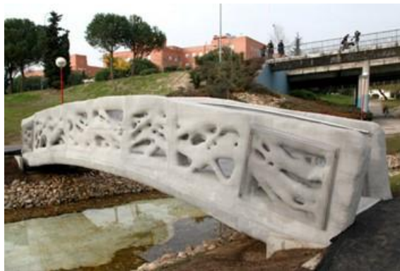
Fig. 21 The first printing concrete bridge by ACCIONA
